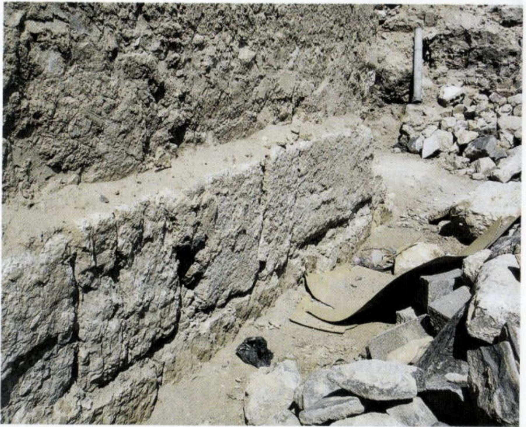
FIG. 68 Roman ashlar blocks running east–west in north wall, middle courtyard, Bayt Farhi, 2006 (S. Weber).
